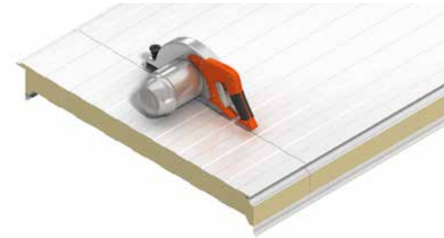
Cut the bottom metal skin using the appropriate tool
