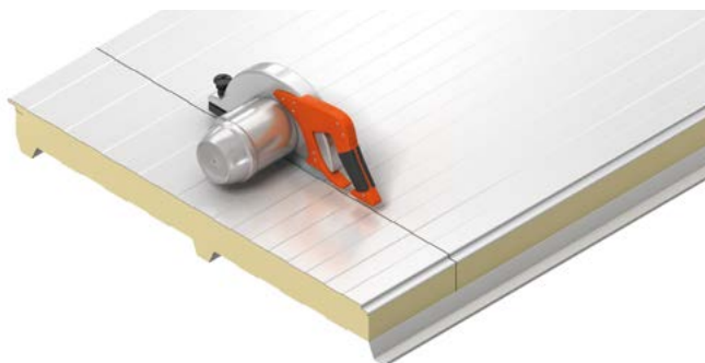
Cut the bottom metal skin using the appropriate tool
