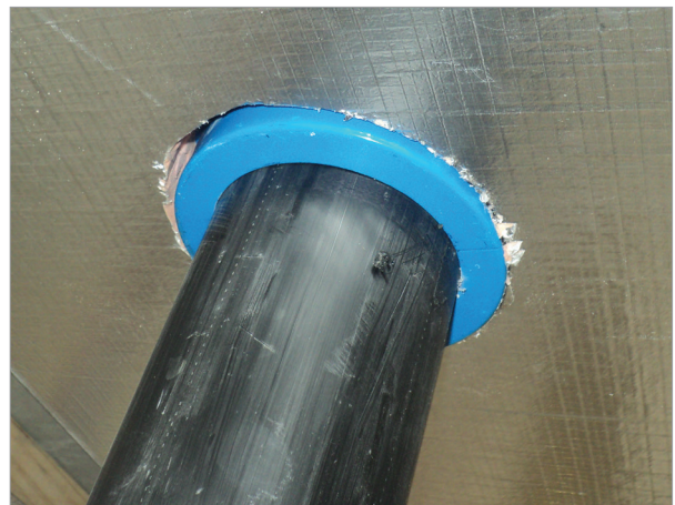
Figure 7. Penetration example - Kingspan Kooltherm® K10 G2 Soffit Board installed tight around the fire collar and HDPE service pipe.
