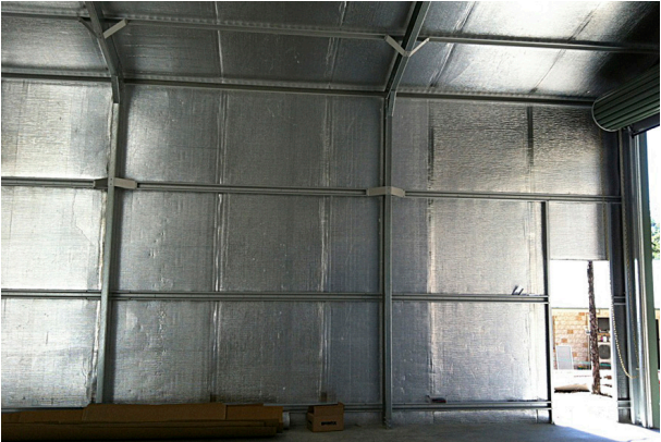
Figure 1. Side elevation of Kingspan AIR-CELL Insulshed® 50 in a metal roof shed.
